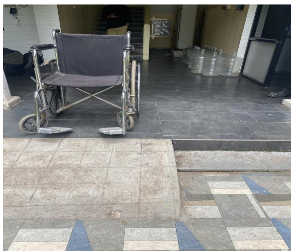
Ramp 3 – Canteen Block
